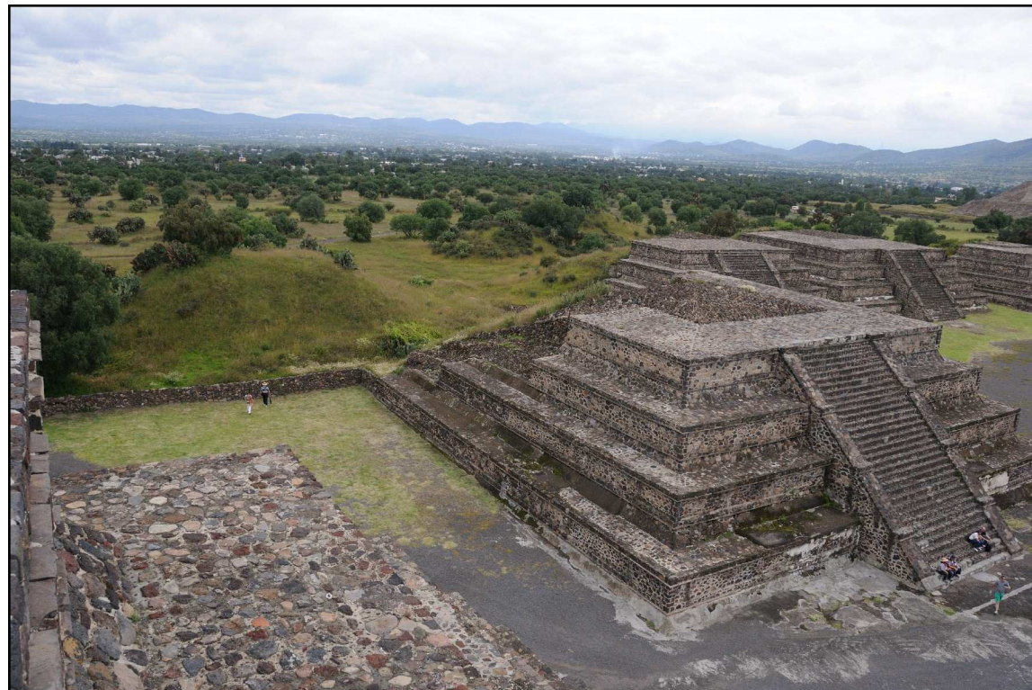
"Restoration in Progress" Aztec City of Teotihuacan, Mexico City
